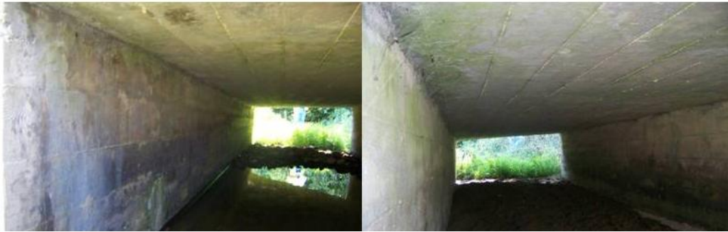
Figure 5: Inner Structure of Box Culvert
